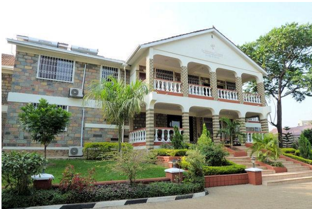
Note solar panels on roof for hot showers.
